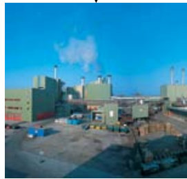
fluidized bed incinerator 4
