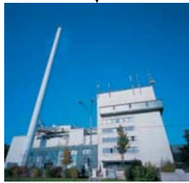
incineration plant Flötzersteig
