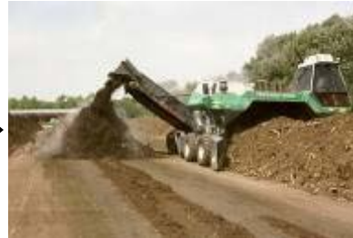
composting plant (starting 1991)
