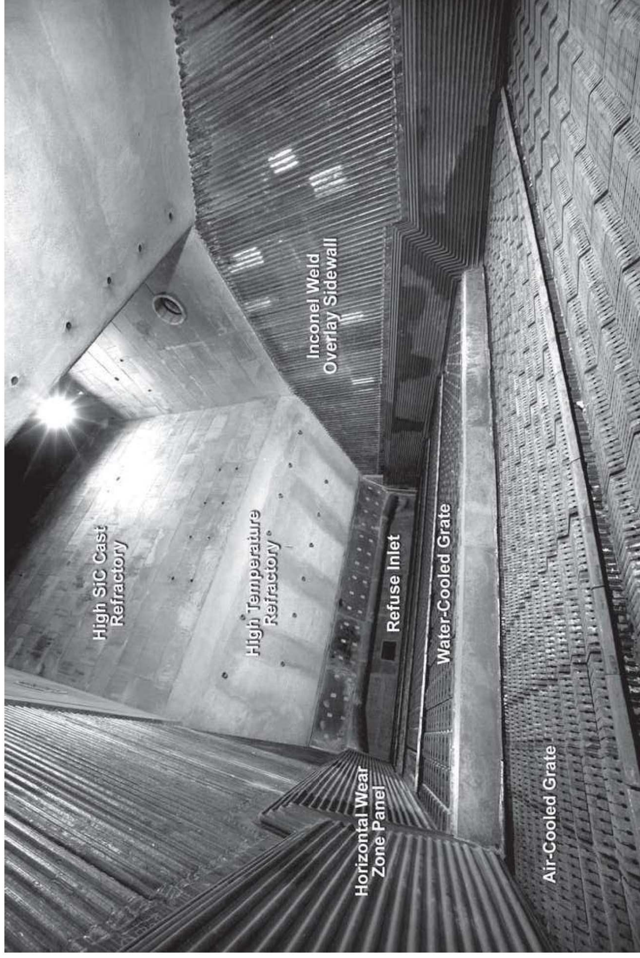
Fig. 7 Corrosion protection and design of a 26 t/h mass-fired unit.
