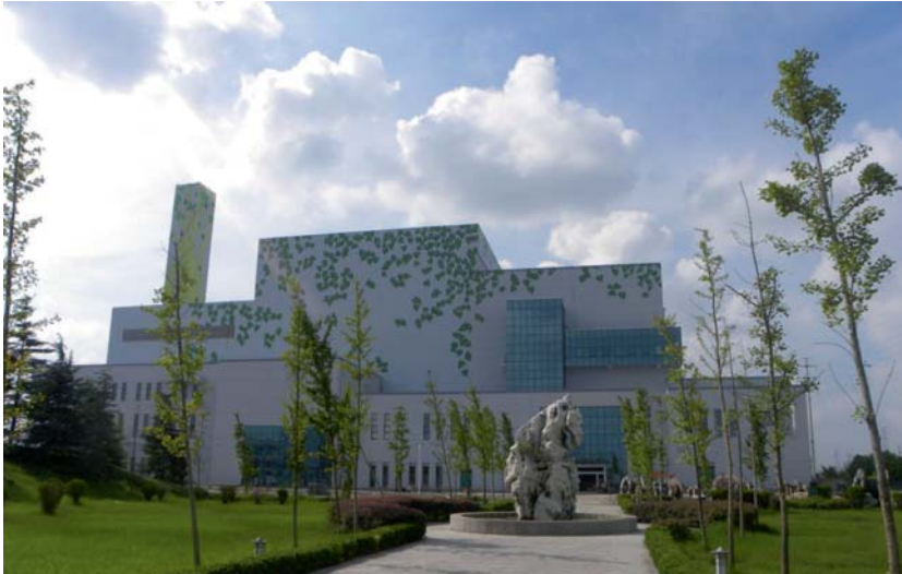
Figure 2: CNTY Hai'an WtE plant (3x250TPD), 15 MWe with WATERLEAU Energize® grate
