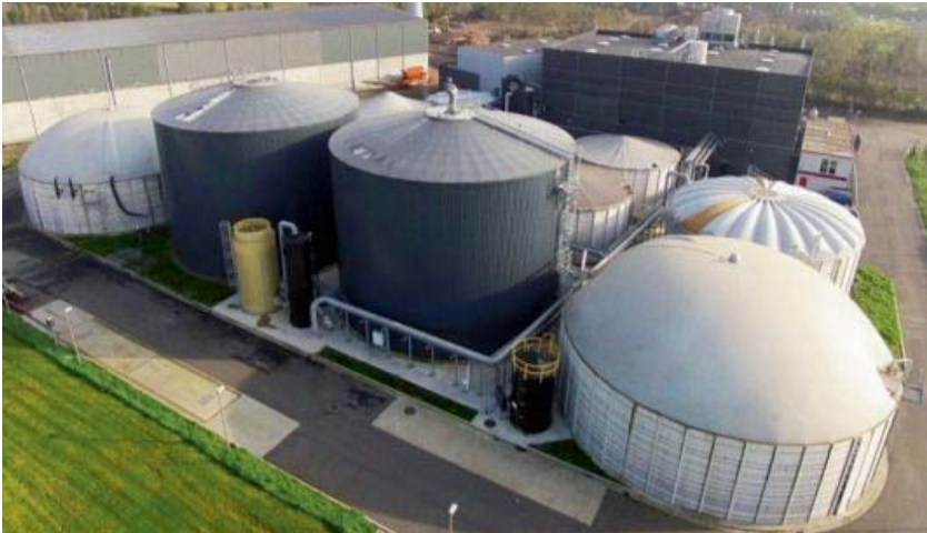
Figure 4: WATERLEAU New Energy Ieper, Biotim® Wet AD plant, 3.2 MWe
