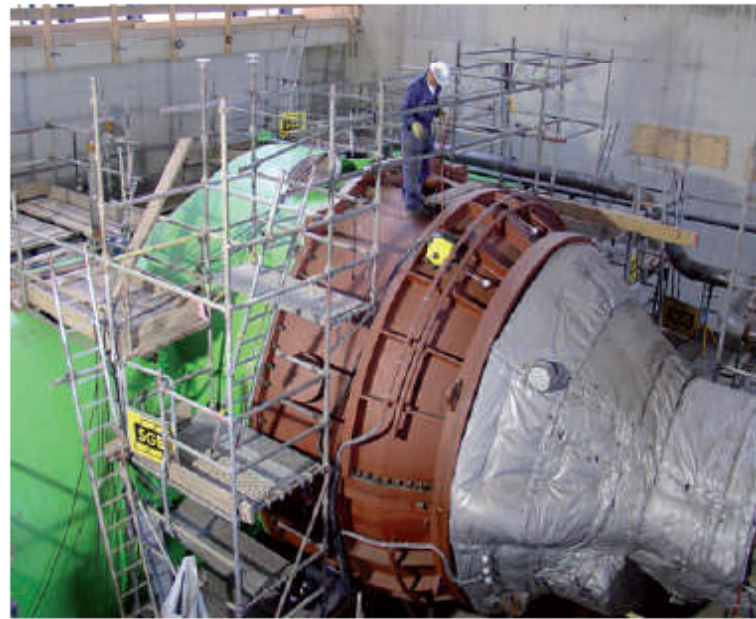
Left: The SST-700 RH installed in the plant, showing noise enclosure (red) over the HP-module, generator and gear.
