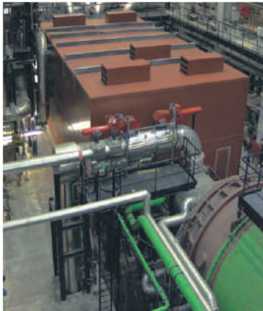
Left: The SST-700 RH installed in the plant, showing noise enclosure (red) over the HP-module, generator and gear.
