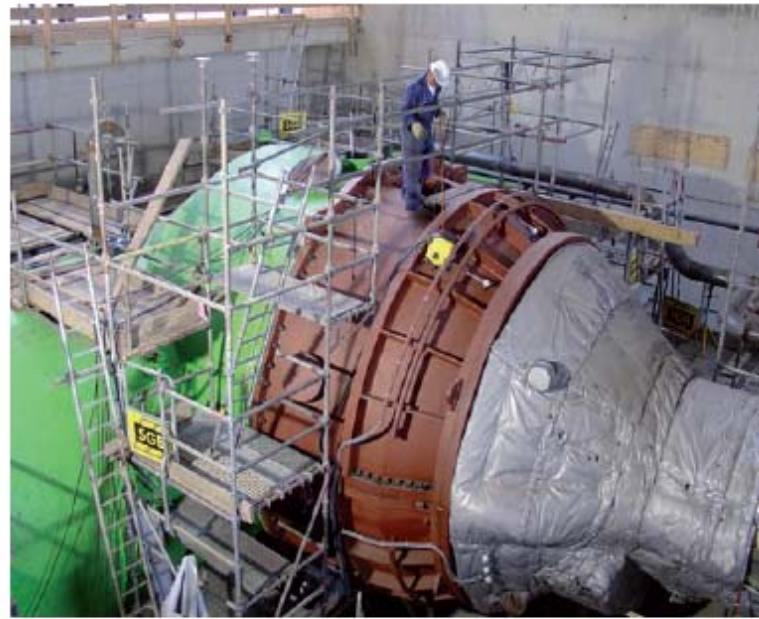
Left: The SST-700 RH installed in the plant, showing noise enclosure (red) over the HP-module, generator and gear. Right: SST-700 LP-module, condenser (green), LP inlet (silver), LP exhaust (brown).
