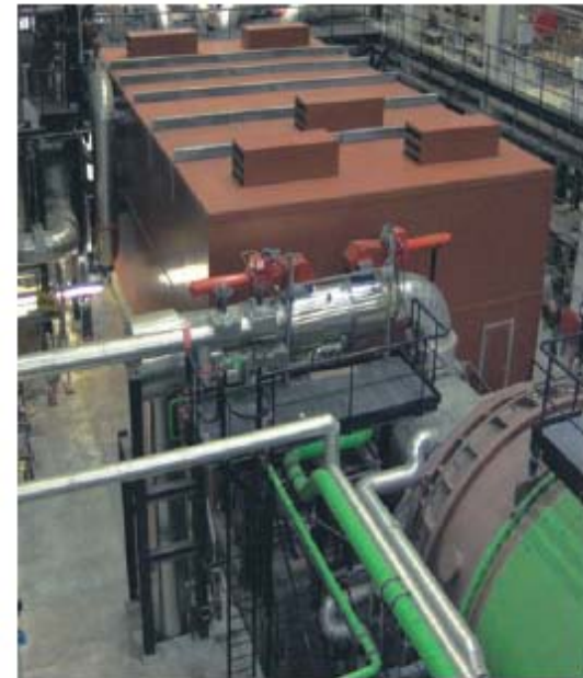
Left: The SST-700 RH installed in the plant, showing noise enclosure (red) over the HP-module, generator and gear. Right: SST-700 LP-module, condenser (green), LP inlet (silver), LP exhaust (brown).
